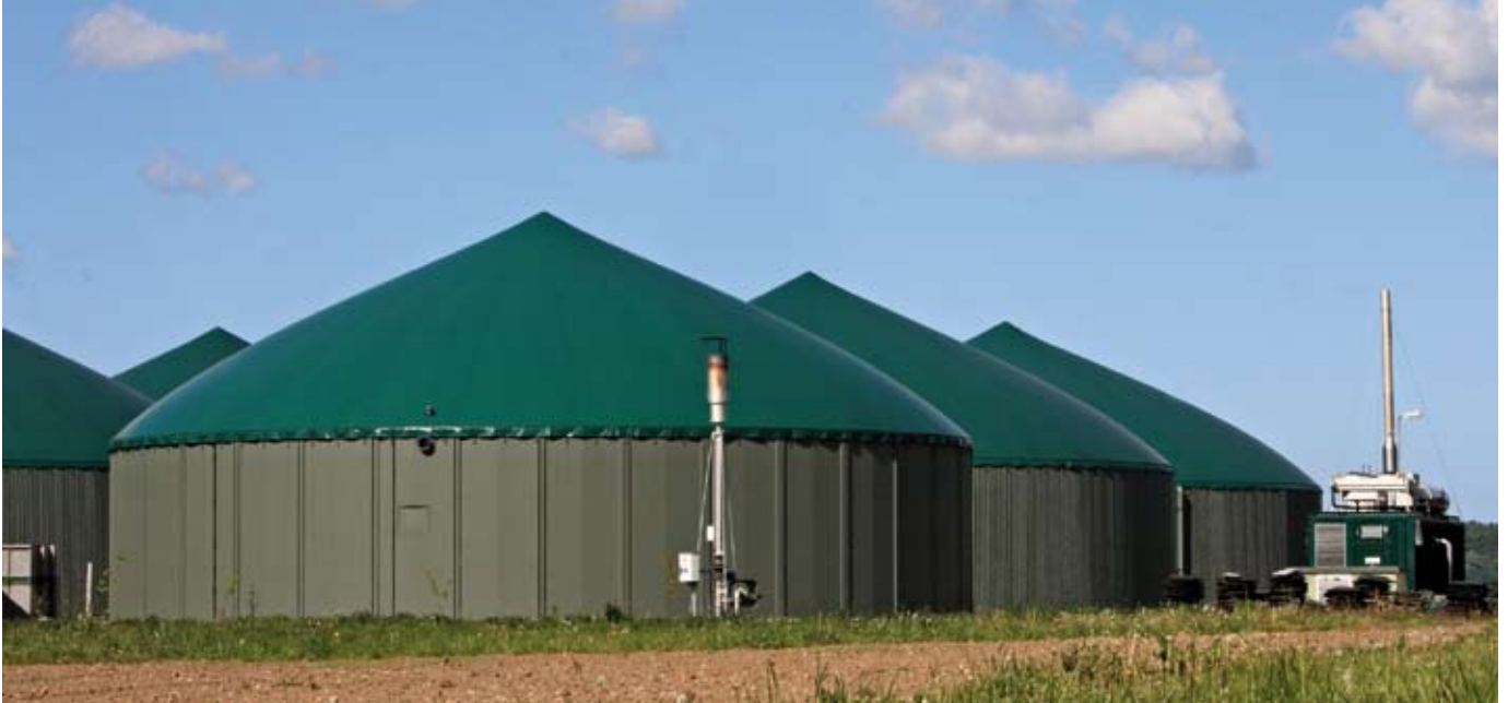
Biogas plants set high valve engineering requirements
